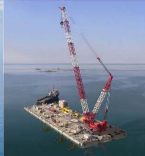
Construction barge Ersai 1 (B, D, WSD)
