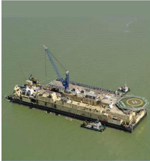
Pipelay barge Castoro 12, assembling (WSD)
